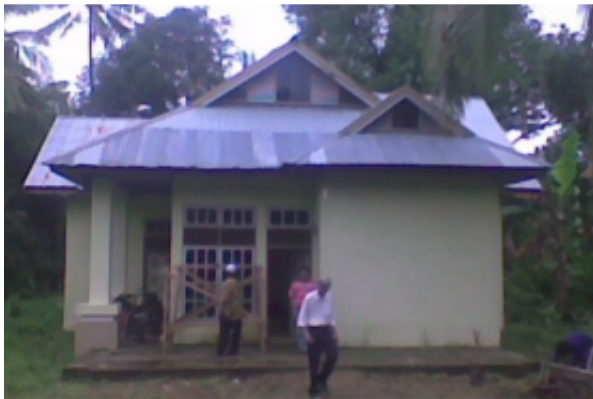
Station Under Construction
