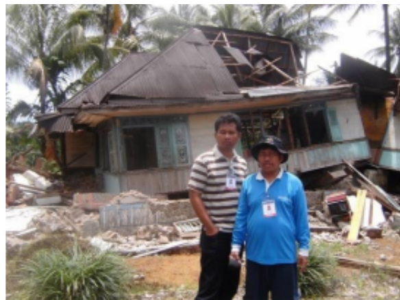
Earthquake Damaged Home
